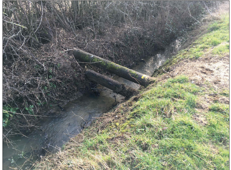
Photo 1: Example of a leaky log jam. Note; to be set a minimum of 450mm off of bed to allow normal flow to continue unaffected.
